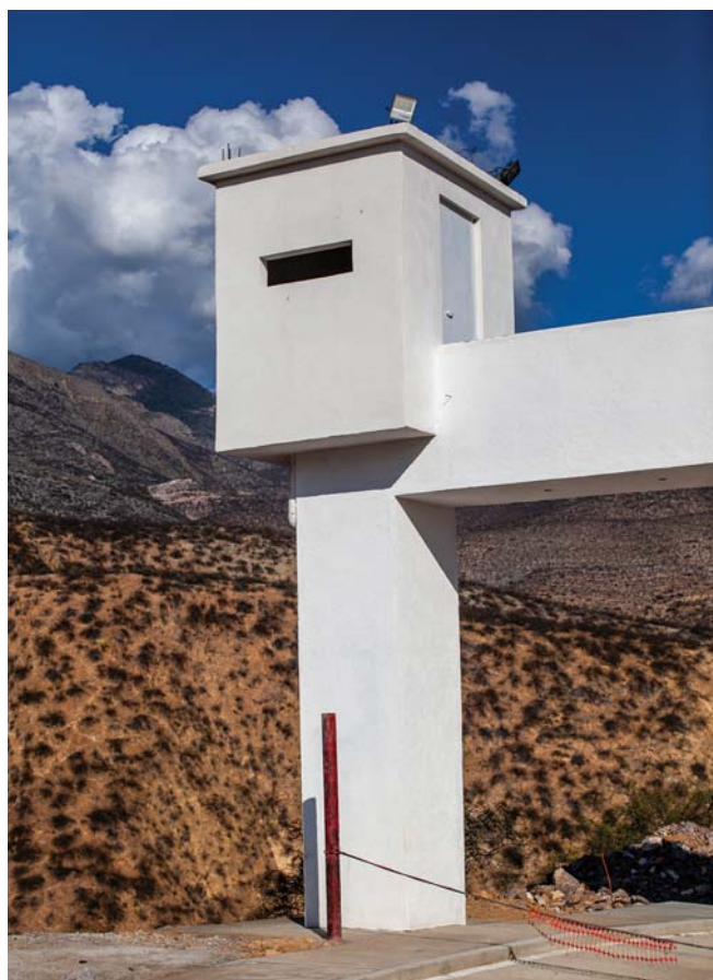
Figure 15 Recently built observation tower and gate on the access way to some of the most productive mercury mines in Queretaro.
